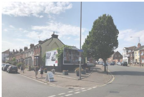
Existing view of corner plot opposite station
