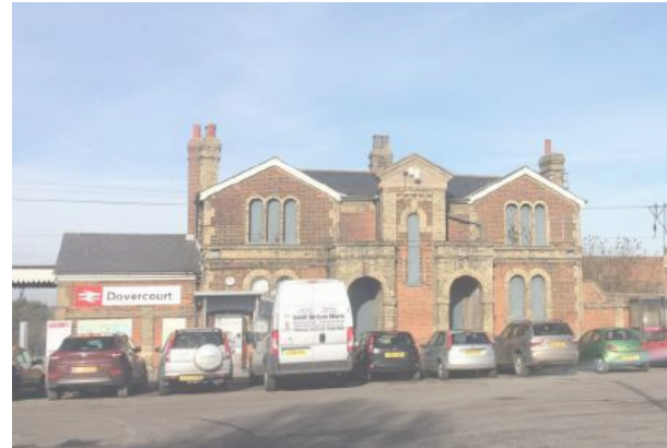
Existing view of train station
