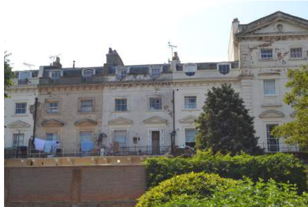
Orwell Terrace properties in a state of neglect, viewed from within Cliff Park
