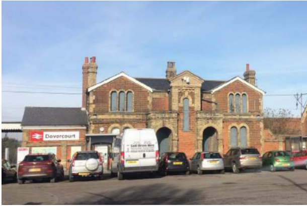
Dovercourt train station
