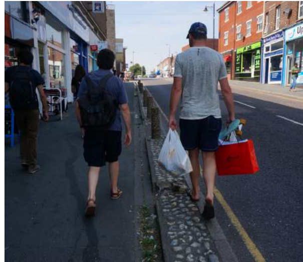
Existing poor quality public realm in Dovercourt
