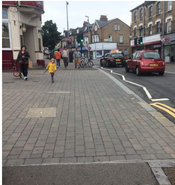
Raised footway level side street entry treatments emphasise pedestrian priority
