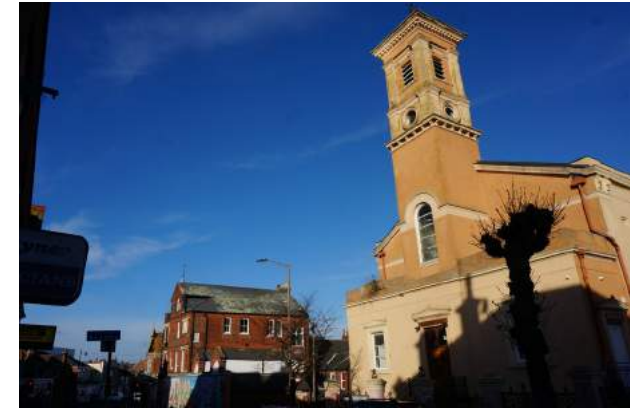
Kingsway Hall, a Grade II Listed building which acts as a local landmark
