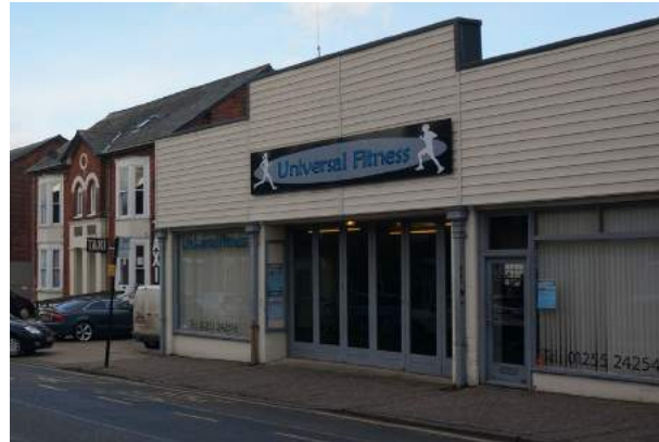
Some existing shopfronts are unattractive and feel outdated
